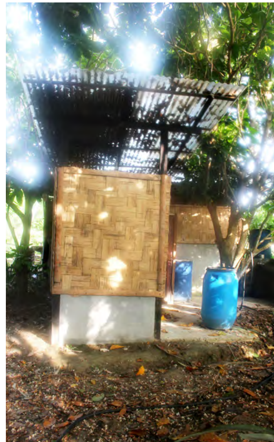
NEW TOILET AND BATHROOM BLOCK
