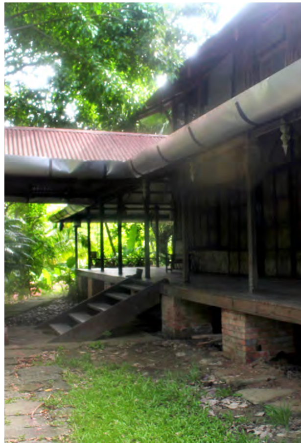
RAINWATER HARVESTING SYSTEM
